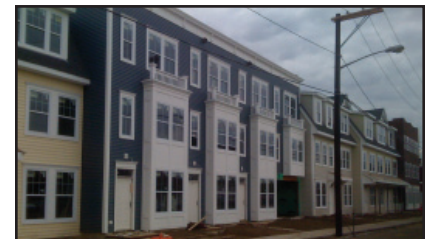
Project under construction
